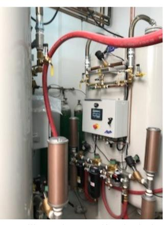
We install a duplex Oxygen generator so by that way we will never have a malfunction in the O2 generator in which it is very essential for the hospital.
